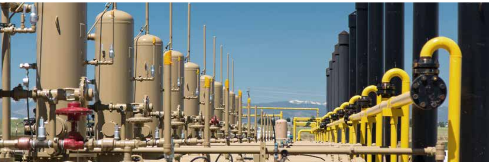
NEWLY ESTABLISHED OIL SEPARATION UNITS ON THE WIND PAD, USA
